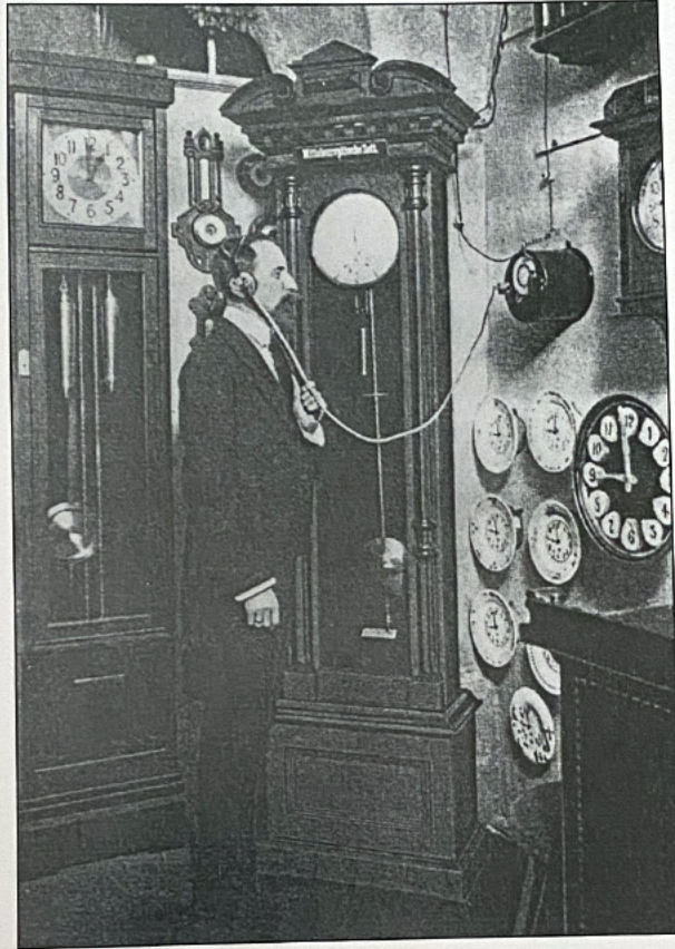
Fig. 34-28. The time service installation at the offices of the German Clockmakers' Journal, which was controlled by Strasser & Rohde's Precision Pendulum Clock.
